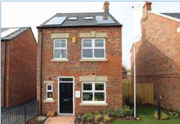
Farndale Housing Development
